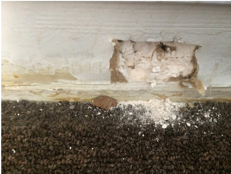
Photo 2: Non ACM white drywall system
