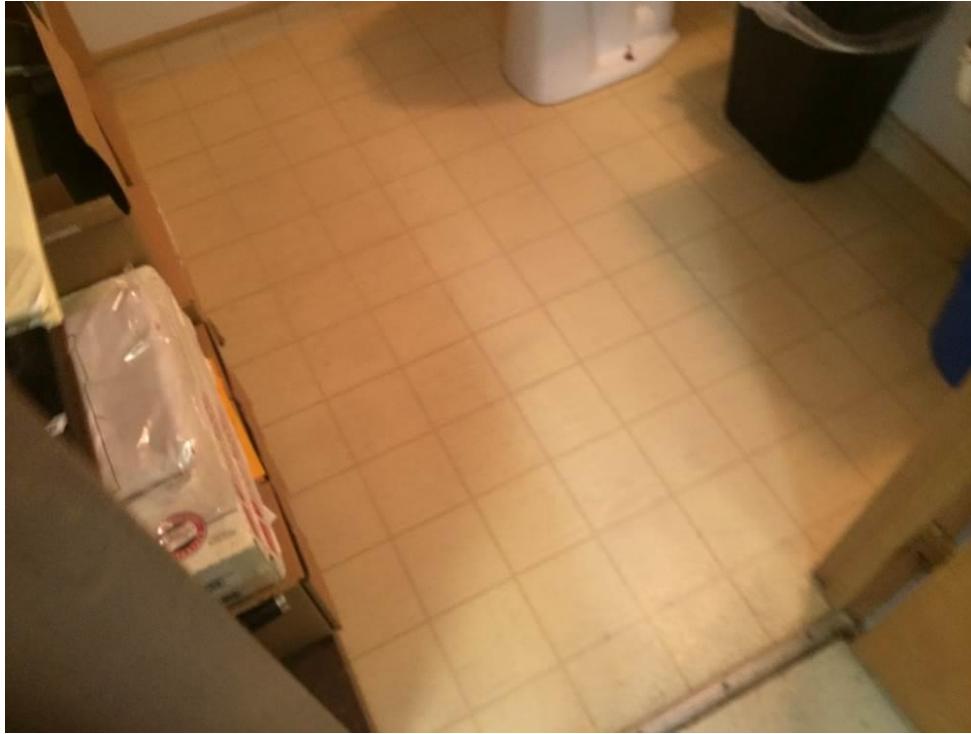
Photo 5: Non ACM yellow linoleum
