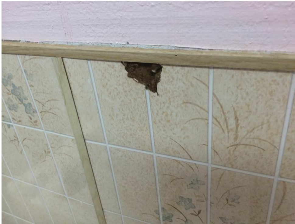
Photo 13: Non ACM yellow wall linoleum
