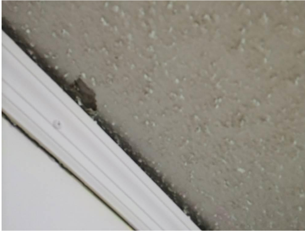
Photo 3: NonACM white popcorn ceiling finish
