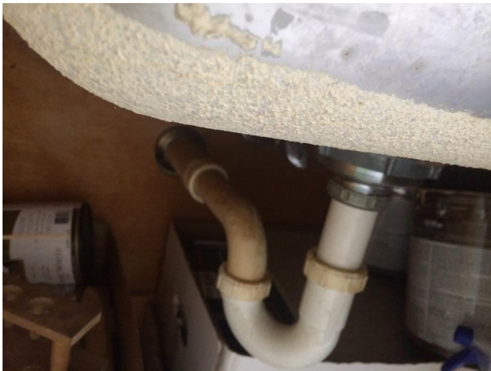
Photo 14: Non ACM white sink undercoat
