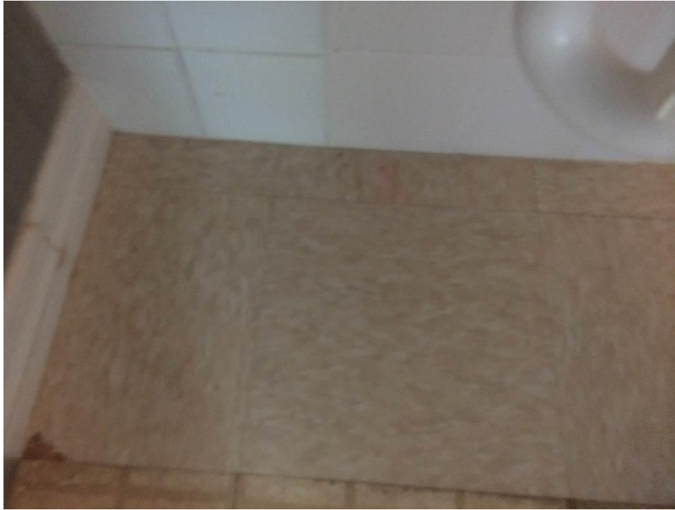
Photo 7: Non ACM Brown 12" VFT
