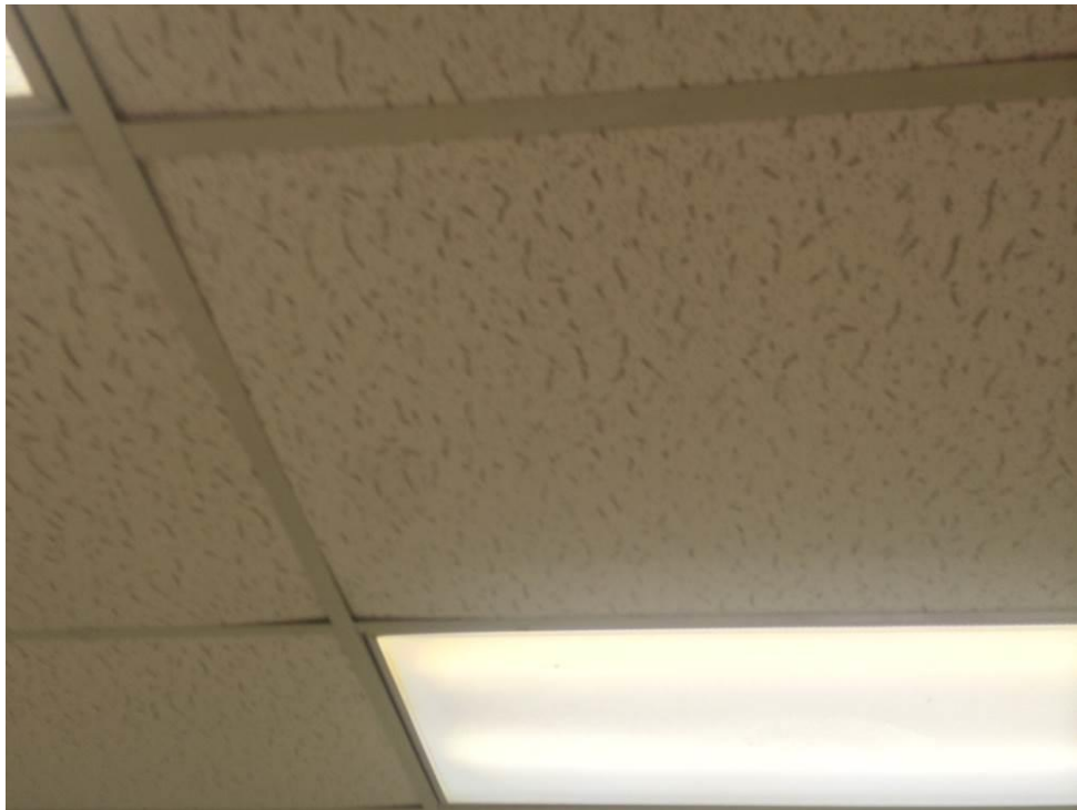
Photo 4: NonACM White 2'x4' ceiling tiles dot furrow
